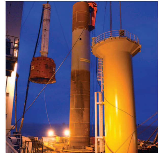
Foundation installation, Swanen.
